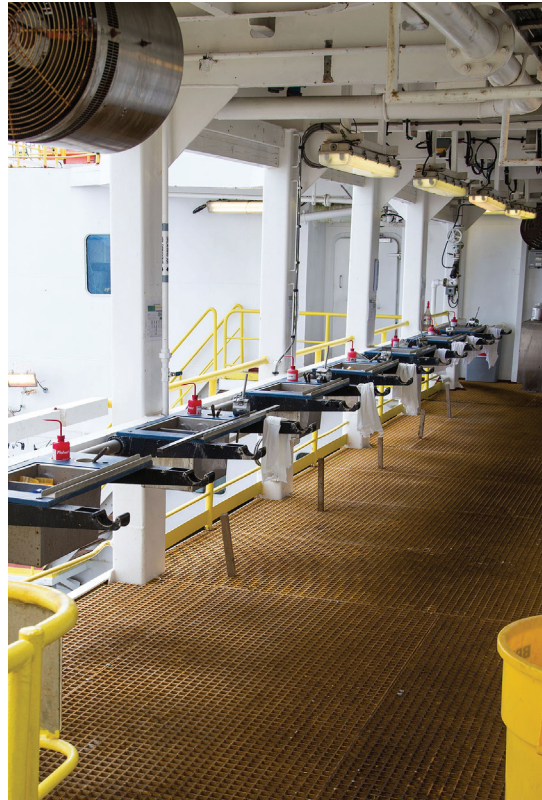
Core-receiving platform on the catwalk awaiting core.
