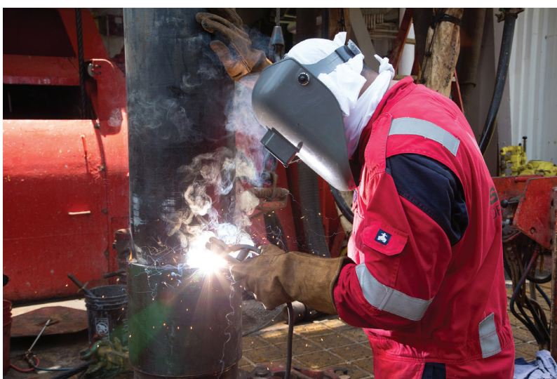
Welding two joints of casing together on the JOIDES Resolution rig floor.
